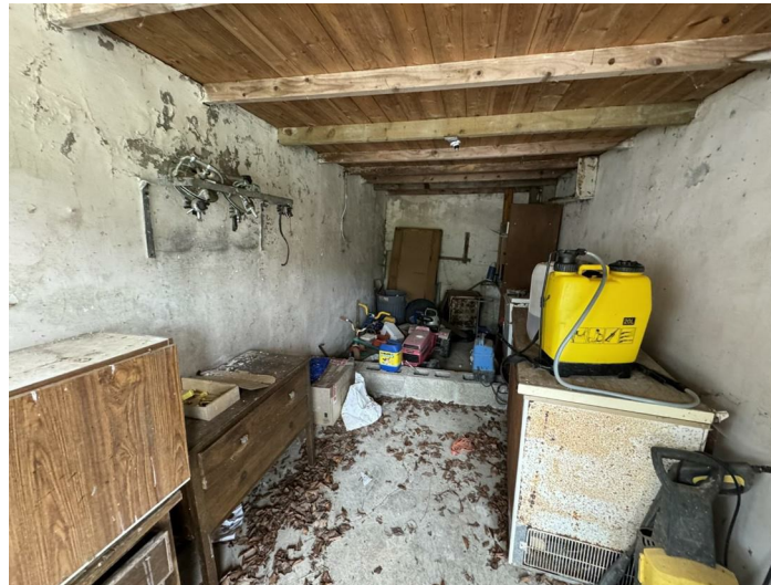
SIDE MUCK STORE with access to adjoining fields.
